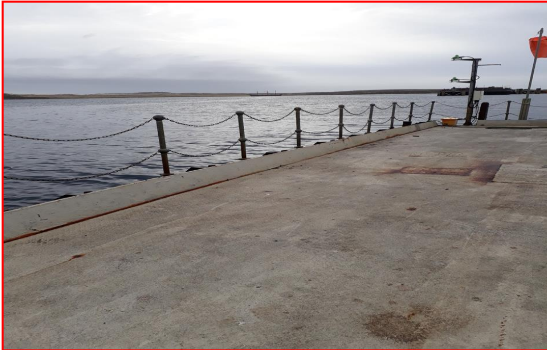
Fig 1: FIPASS RoRo Safety Rails.
