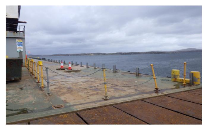
To accommodate new mooring bollards being installed on the northwest barge, the Armco safety barriers have been removed from a significant proportion of the berth face on that barge. We have now removed a critical control measure to reduce the risk of individuals falling into the sea. The deck beyond the stanchions and chains, from the berth face to 2m away from the berth face, has now been designated as a lifejacket zone.
